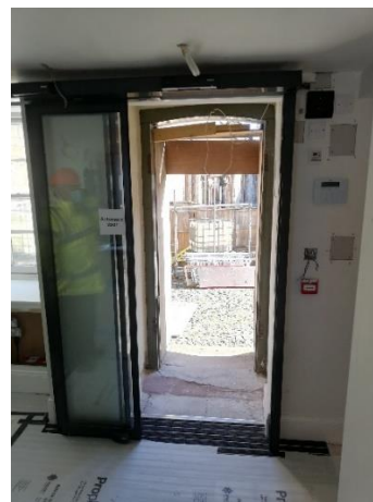
The new sliding entrance doors
