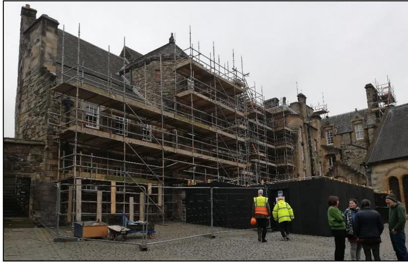
King's Old Building shrouded in scaffolding – HES works on roof, wall and widnows
